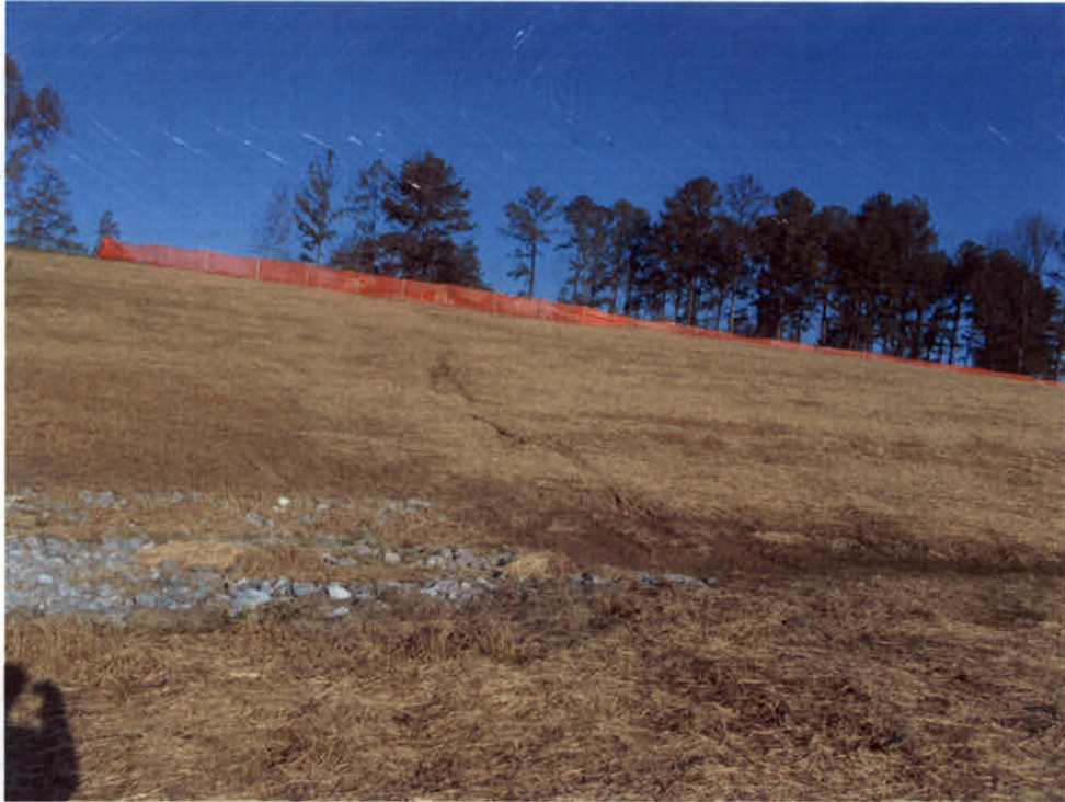
Erosion Rills on Slope
