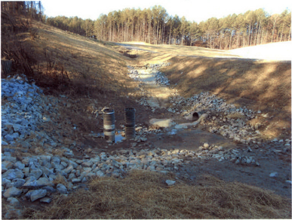
Sediment Basin 1 Discharge Point
