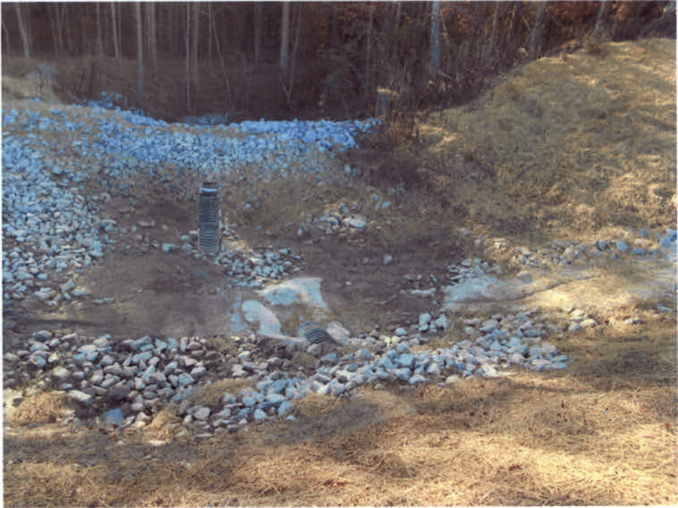
Sediment Basin 1 Discharge Point
