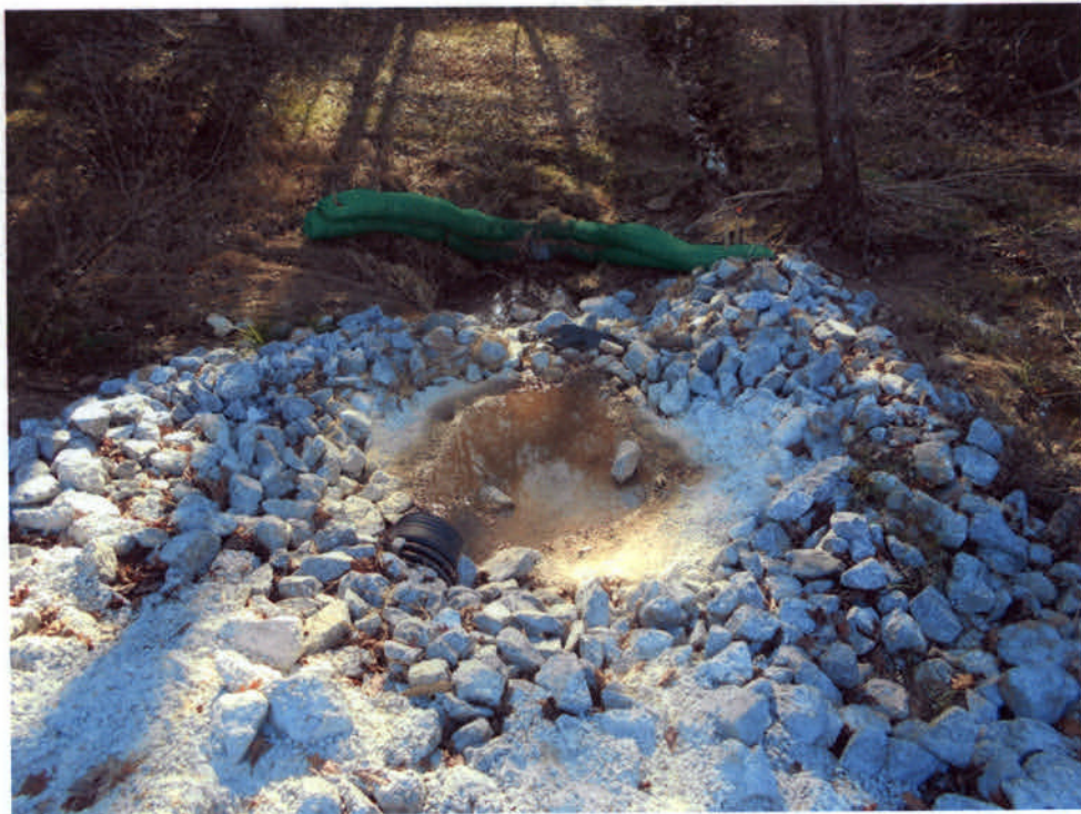
Sediment Basin 2 Discharge Point
