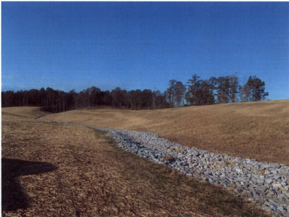
Rip-Rapped Drainage Ditch
