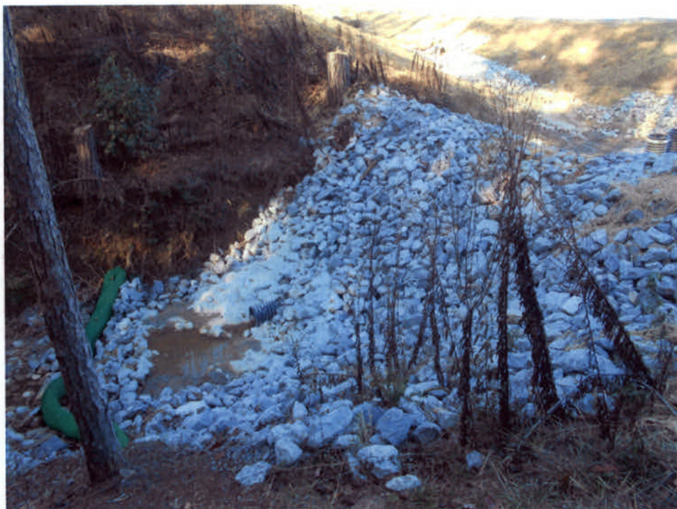
Sediment Basin 1 Discharge Point
