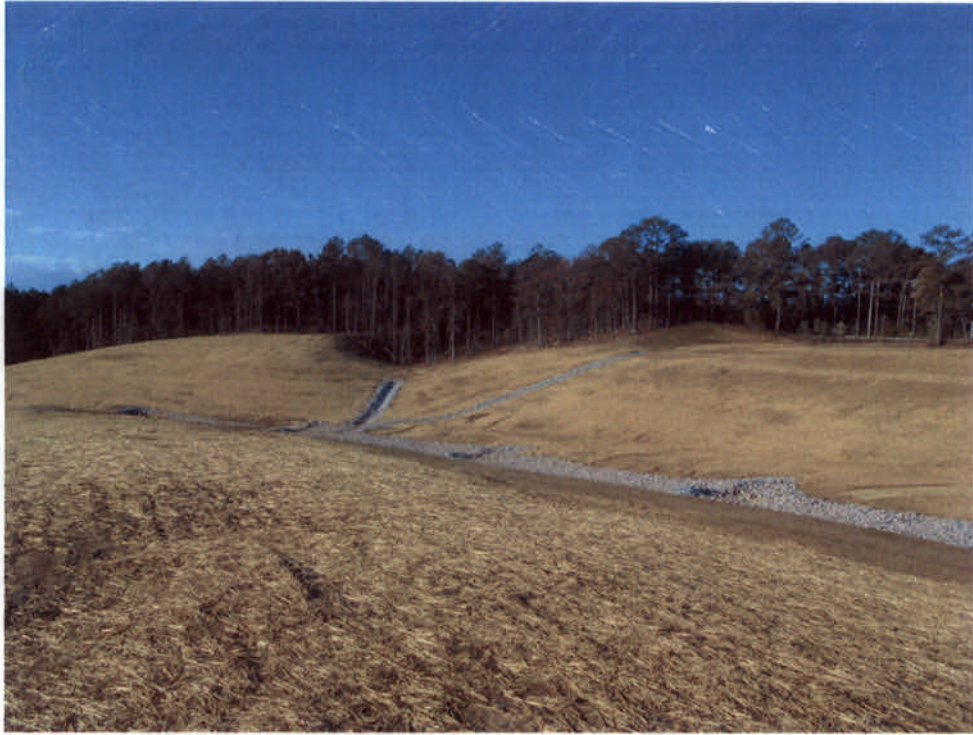
Rip-Rapped Drainage Ditch with Check Dams
