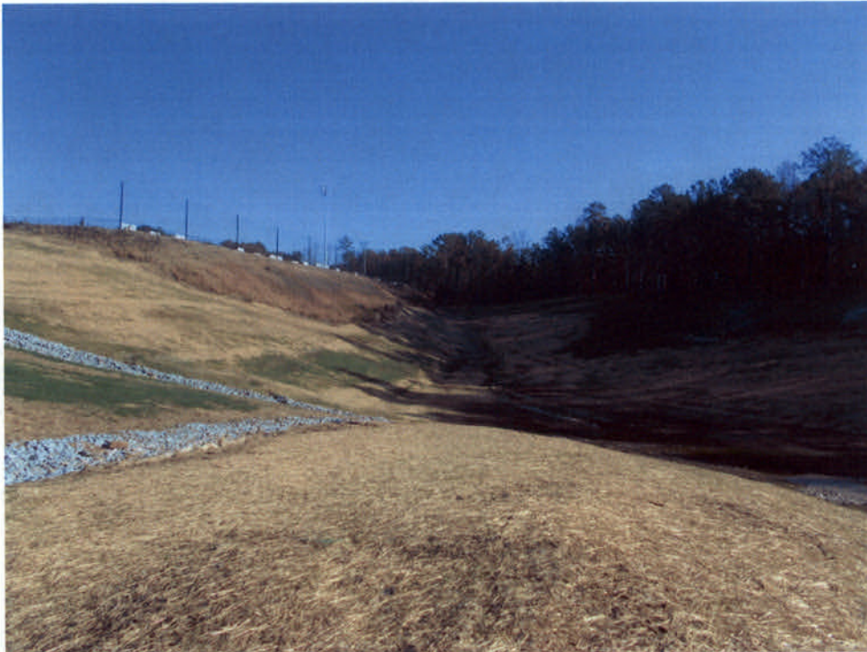
Drainage to Sediment Basin 2
